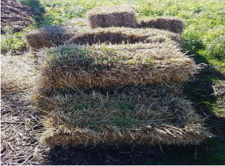
Fig 5: Straw bales stored in lay down area off of Gosling Rd in open area need To be covered. Viewing east. (6-18-19).
