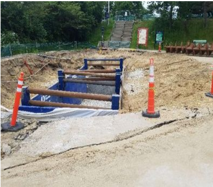
Fig 7: McCourt finalized the jacking pit in "A" lot. Viewing south. (6-18-19)
