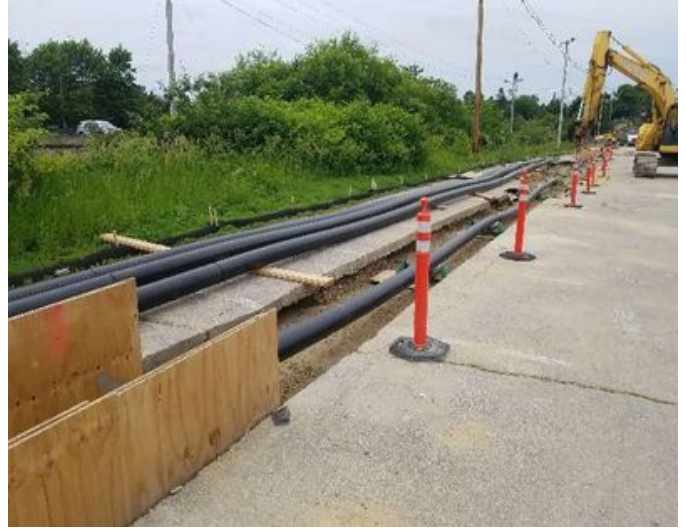
Fig 6: McCourt installing pipe and duck bank in "A" lot. Viewing south. (6-17-19).
