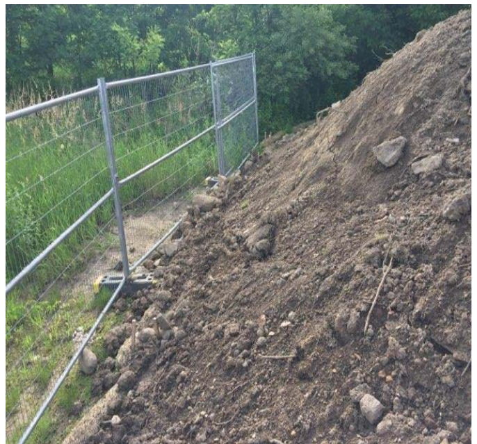
Fig 8: Soil stockpile in Waterworks Rd laydown area overtopped the Straw wattle. Viewing east. (6-17-19).
